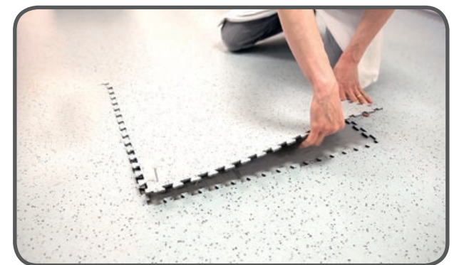
Damaged tile out / New tile in
